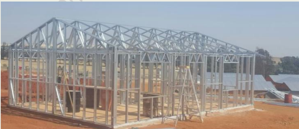
Plumbing & Electrical installation commences after first frames are installed
